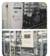
Water treatment facilities
